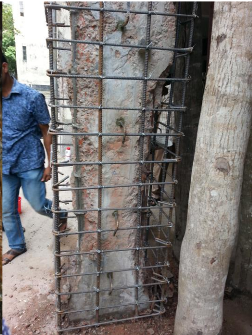
Photo-4: columns during retrofitting phase
