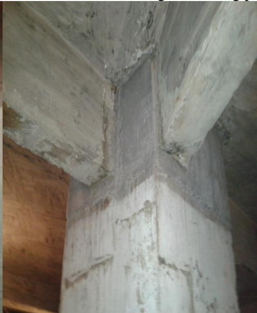
Photo-6: Column after retrofitting
