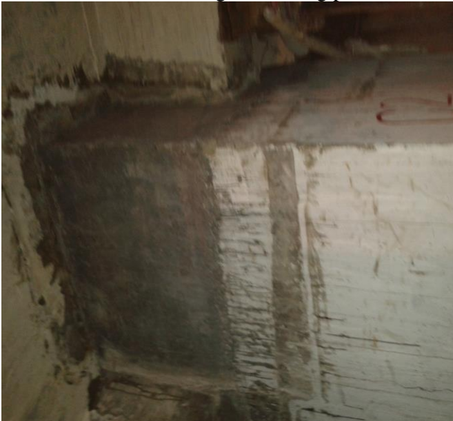
Photo-5: Column after retrofitting
